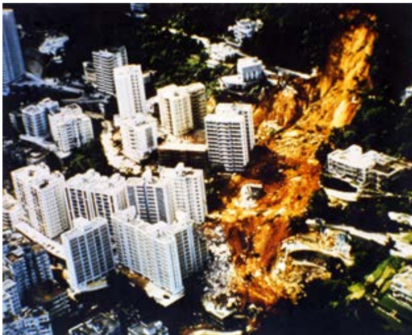
Po Shan landslide on Hong Kong Island in 1972.
